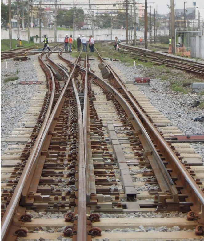
CPTM Sao Paulo T/O 60E1 500-1:14 type 3 1600/1000mm gauge with moveable obtuse crossing
