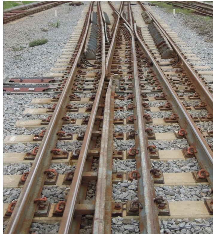
CPTM Sao Paulo T/O 60E1 500-1:14 type 3 1600/1000mm gauge with moveable obtuse crossing
